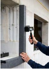
5. Fit the upper blaugelb Trio**therm**\* profile. Seal the butt joints of the side profiles using blaugelb Hybrid Polymer Power Fix.
