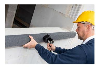
The applied blaugelb Hybrid Polymer Power Fix works immediately as an ancillary fixative. Its high initial adhesion means that the profile adheres immediately at the intended position. Slight adjustments to its alignment will be possible for up to about 20 minutes after applying to the anchor base.
