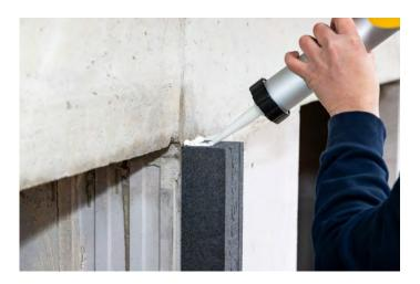
6. Position the blaugelb Trio**therm**\* profile and press it firmly onto the anchor base and the side profiles.
