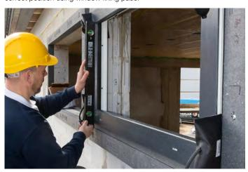
2. Note the fixing specifications / fixing spacings (**Appendix III**) when screwing the window frame into the blaugelb Trio**therm**\*. It is essential that you observe these. Use **only** the blaugelb Frame screws FK/ZK-T30 7.5 mm to fix the window elements directly in the blaugelb Trio**therm**\* profile. Do not pre-drill the blaugelb Trio**therm**\* profiles.
