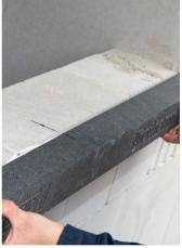
2. Press the prepared blaugelb Trio**therm**\* profile firmly against the anchor base, making sure it remains in the marked position. The profile can be pressed on firmly using a hammer with rubber attachment.
