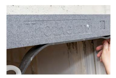
Once the upper tape has been fixed in position, use the blaugelb 40x60x10 mm Spacer Block (item no. 0416311) to mark the space that the upper tape needs in order to expand.
