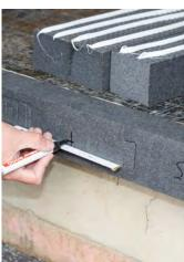
Always work on the basis of 200 mm from the inside corners, except in the case of the lower profile.
