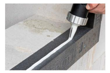
4. The window frame is then fitted into the frame aperture using the blaugelb Sill Connection Profile EPS.
