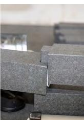
In the area of the dovetail joint a screw connection (to the profile above) must be made at a distance of 100 mm from the joint, regardless of the usual fixing spacings.
