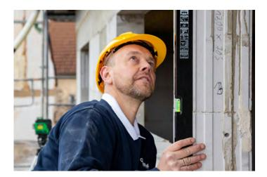
The surfaces of the anchor base must be checked for flatness and vertical and horizontal alignment. Make allowance for centre line tolerances and masonry tolerances.
